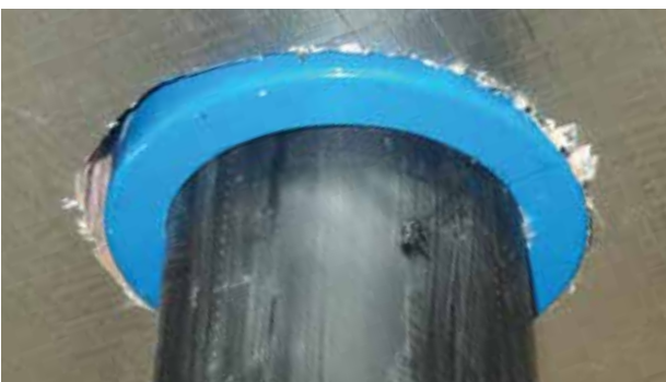
Figure 7 Penetration example - Kingspan Kooltherm® K10 G2W White Soffit Board installed tight around the fire collar and HDPE service pipe.
