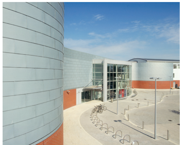
Project: Gloucester Leisure Centre
