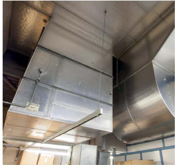
Ductwork fabricated from The *Kingspan KoolDuct*<sup>®</sup> System can reduce air-leakage rates to a fraction of those typical of rectangular sheet metal ductwork. Recent research from Sweett (UK) Limited has revealed that this can lead to “whole life” HVAC savings of over 25% compared with traditional galvanised sheet metal ductwork.
